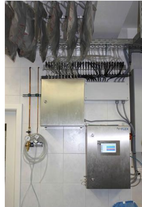
Fig. 6: fix installed gadget
